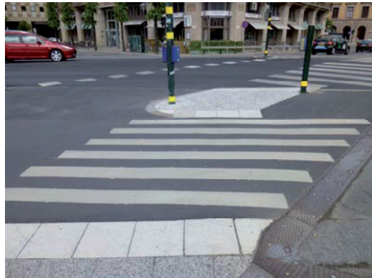
Figure 3. Example of diagonal crosswalk.
