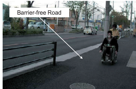
Fig. 4. Overview of Barrier-free Road.
